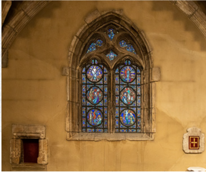
A condition called 'shadowing', which reveals outlines of otherwise hidden concrete block construction, has appeared along walls with exterior exposure. Water staining is visible below the window.
