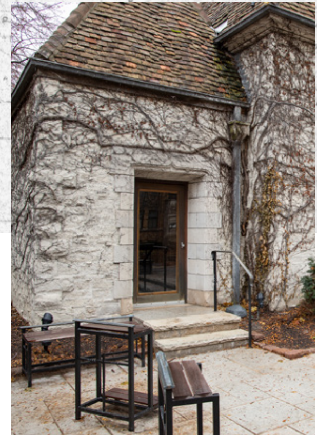
Technology enhancements will provide improved Chapel security and access control.
