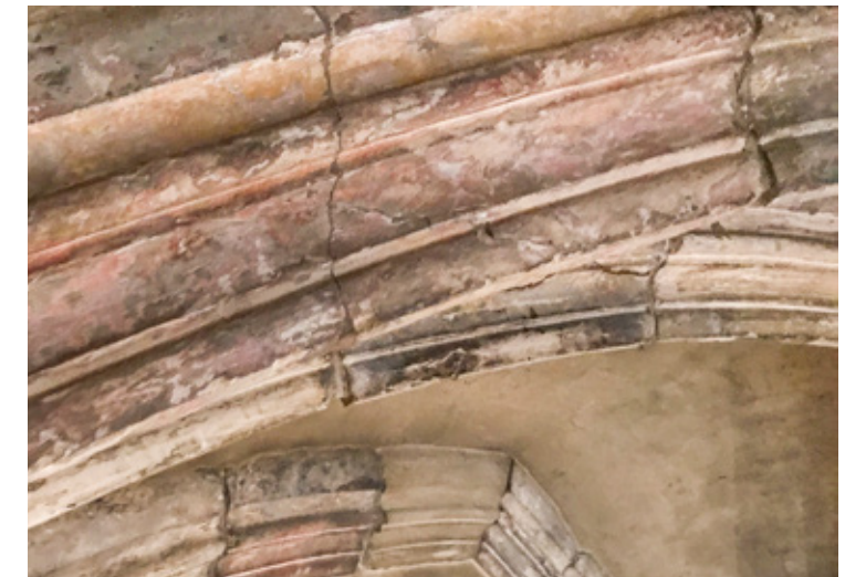
Certain areas of the interior stonework have remnants of historic paint. Examples of original Medieval polychrome painting on stone is rare. Our lab analysis work will look to identify if these are historic paint surfaces indicative of the time period.
