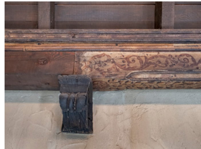
When the chapel was reconstructed on the Marquette campus new wood was added to the historic wood in order to extend the size of the Nave.
