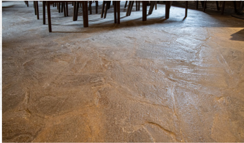
Bluestone flooring installed during the 1966 Chapel reconstruction will be salvaged and reused as part of the proposed new radiant floor heating system.
