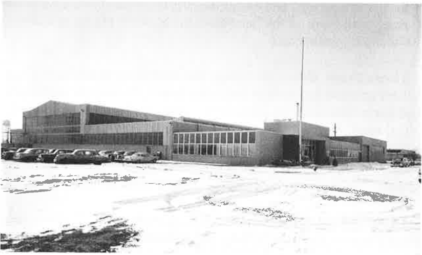
Durethene plant at 7001 West 60th Street
