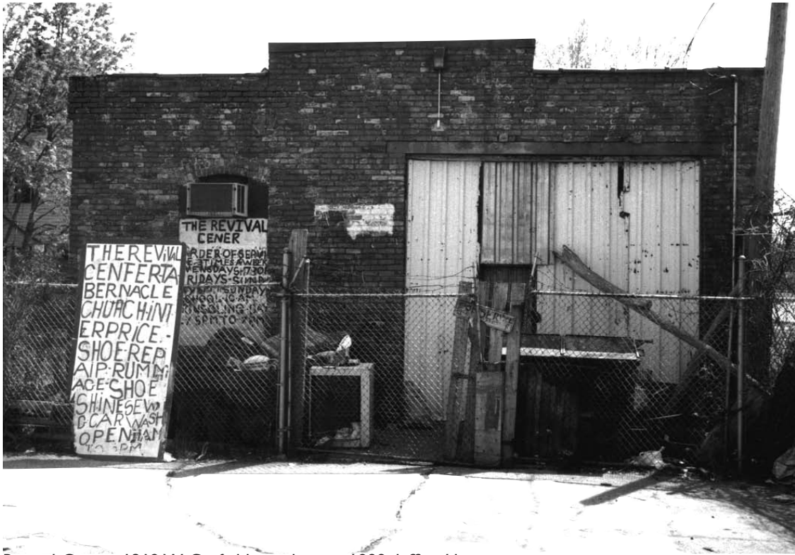
Revival Center, 1312 W. Garfield, north view, 1999. Jeffrey Hayes.
